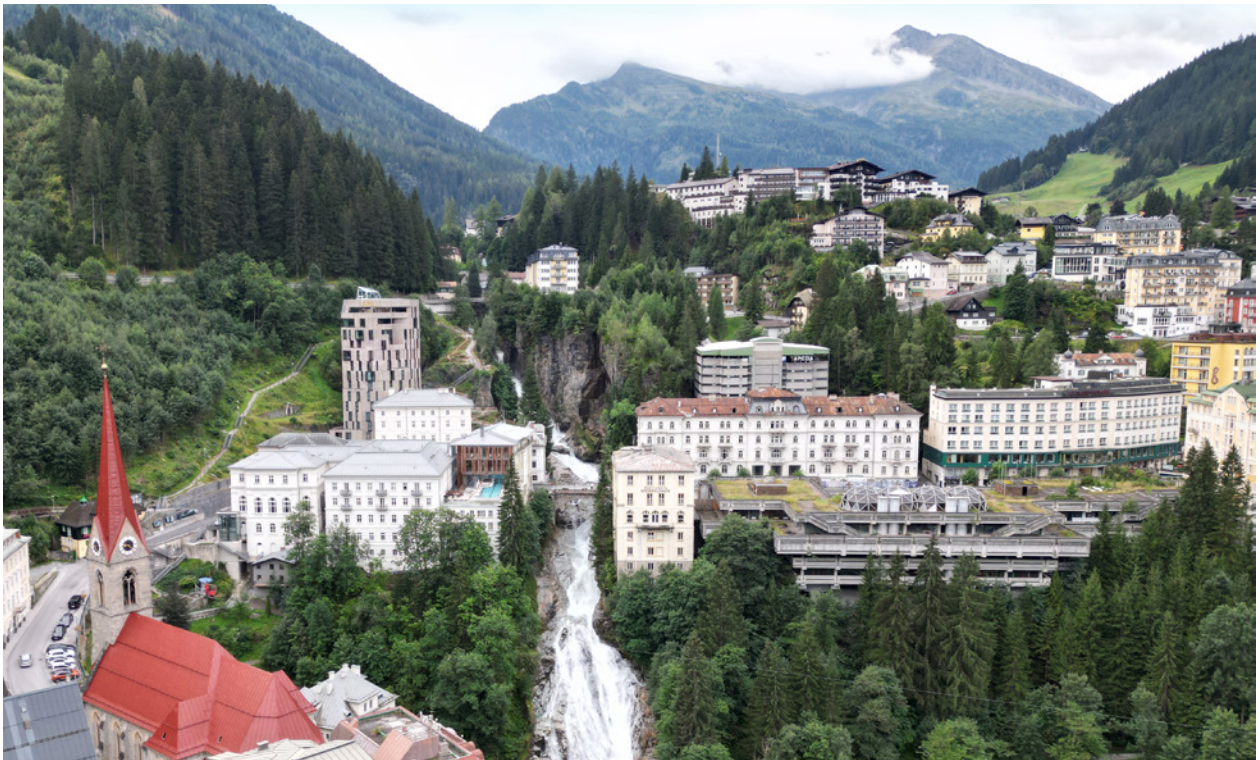
BWM_Bad Gastein_Hotelensemble overview_09_23©BWM Designers & Architects_EduardoGellner
